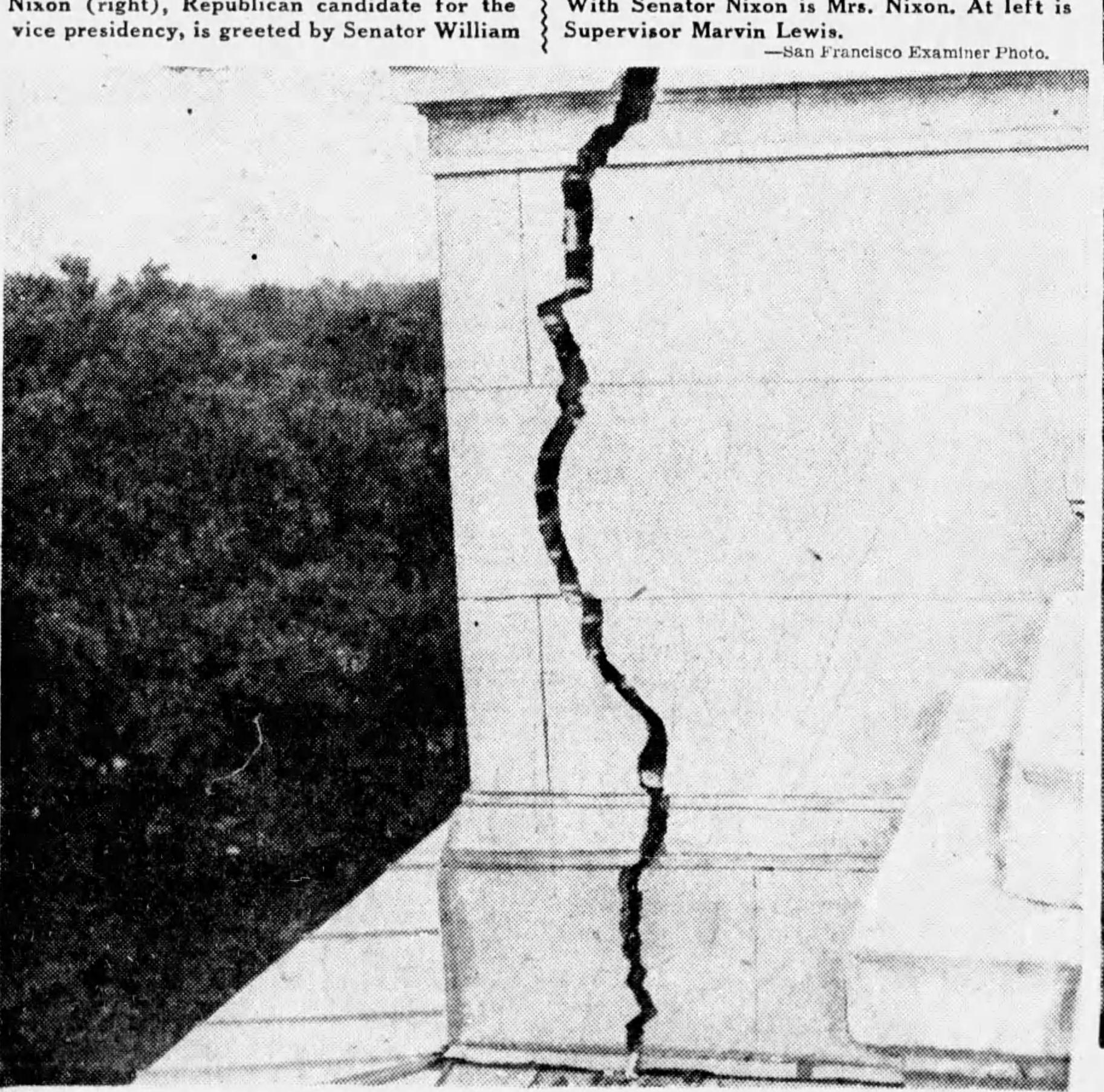
QUAKE DAMAGE - Here is a { County Courthouse at Bakersfield, which was view of the "hanging parapet" on the Kern | cracked by two earthquake shocks yesterday.
